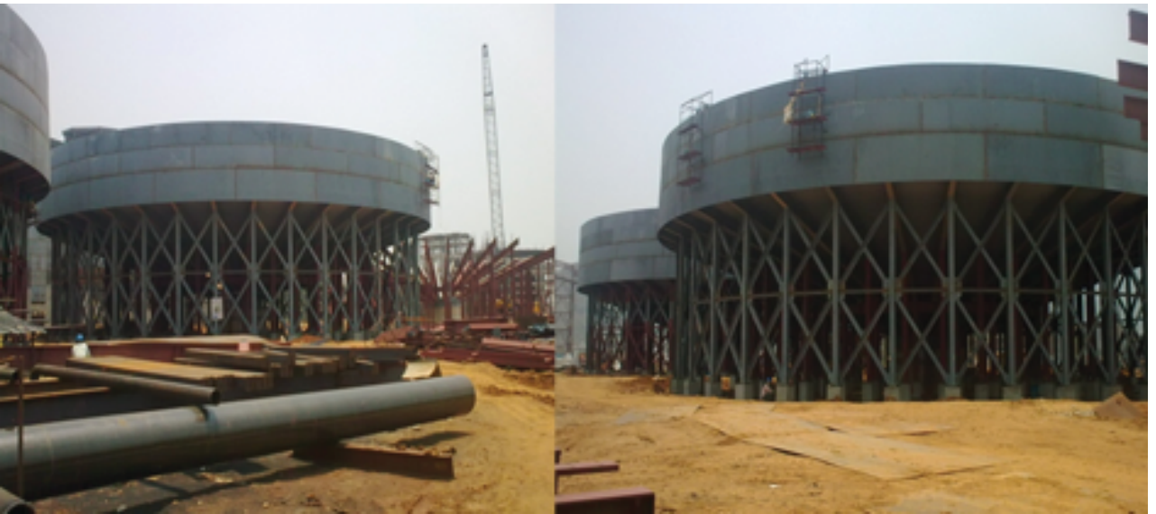
FAB. & ERECTION OF HST TANK AT ANRAK ALUMINIUM – VIZAG
