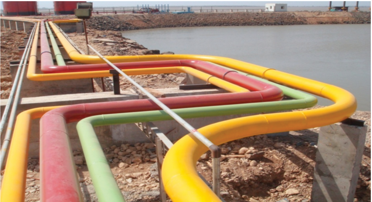
GAS LINE PIPING WORK AT GPPL RAJULA
