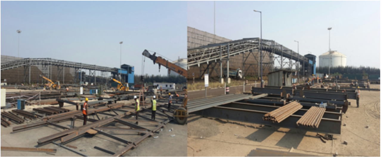
FABRICATION OF CONVEYOR STRUCTURE AT ADANI PORT PVT LTD. . DAHEJ
