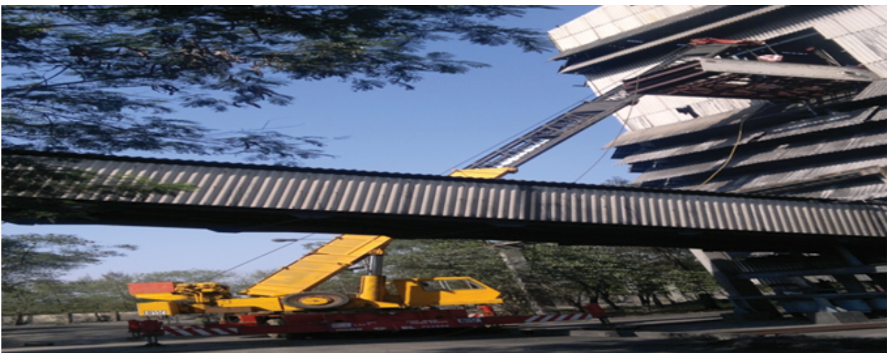
VIBRATING SCREEN ERECTION AT BIRLA CELLULOSIC. KOSAMBA
