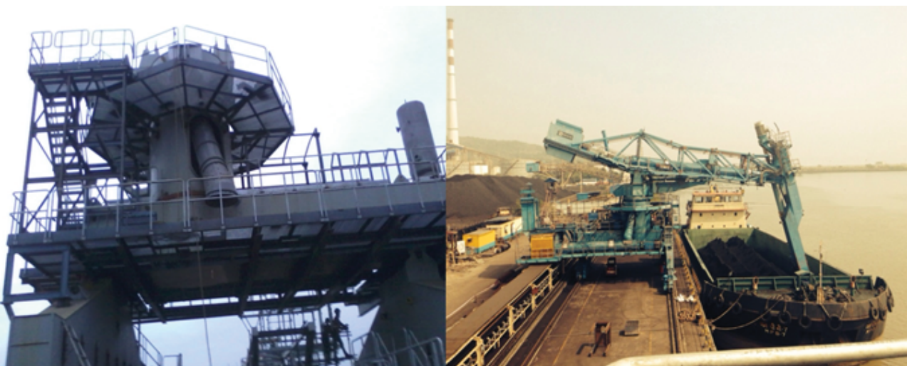
ASSEMBLY, ERECTION & COMMISSIONING OF SCREW TYPE SHIP UNLOADER AT TPCL, MUMBAI
