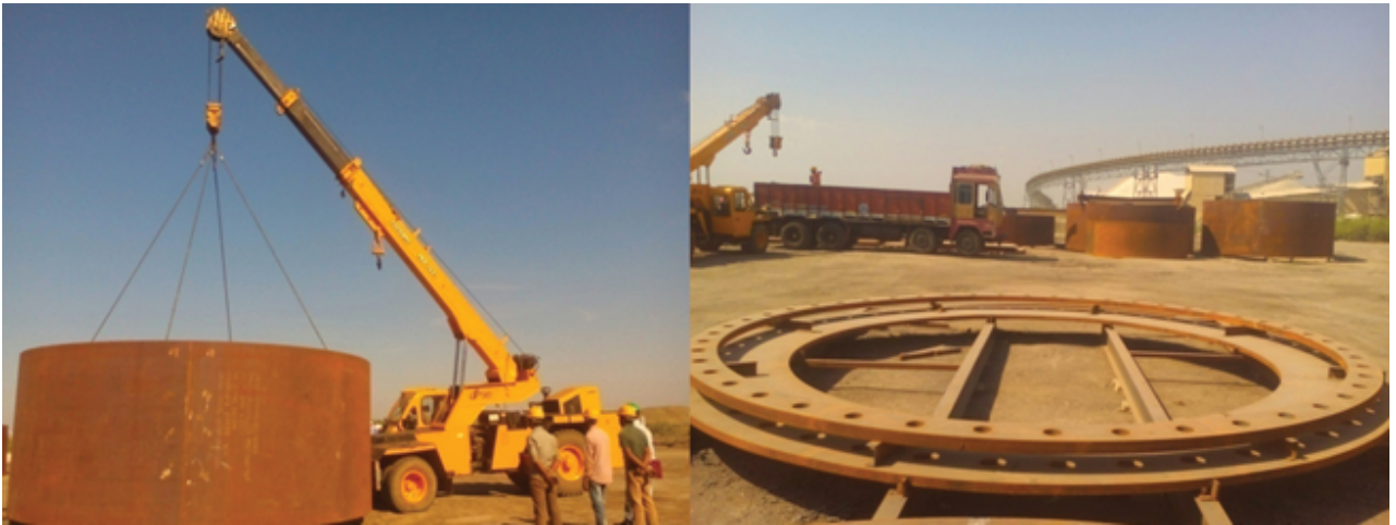
FABRICATION OF VERTICAL KILN AT NIRMA LTD. - BHAVNAGAR
