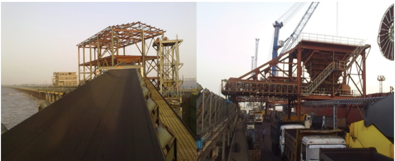
LONG CONVEYOR & MOBILE HOPPER AT ADANI DAHEJ
